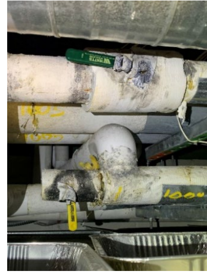
IMPROPER PIPE INSULATION
