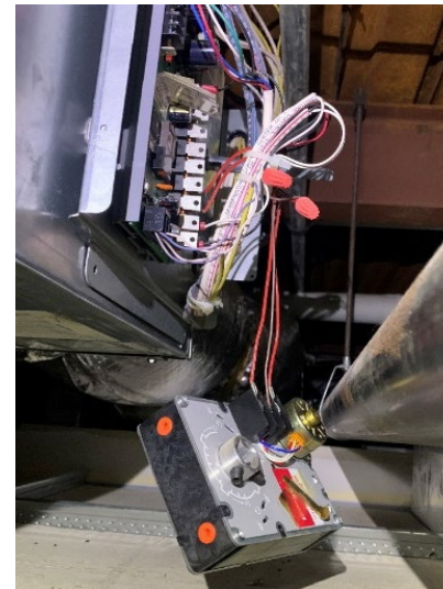
FAILED VAV ACTUATOR
