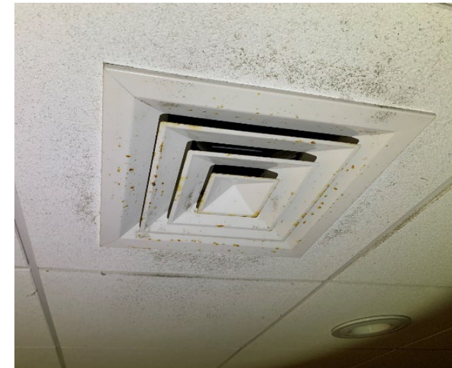
RUST AND CONDENSATION ON DIFFUSER
