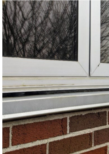
Missing Sealant
