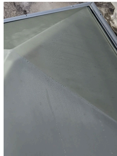
Skylight Condensation Build Up
