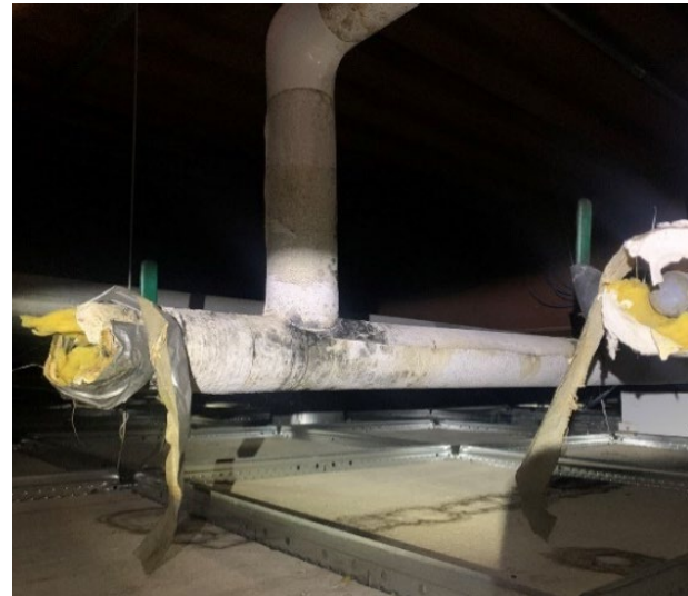
IMPROPER PIPE INSULATION
