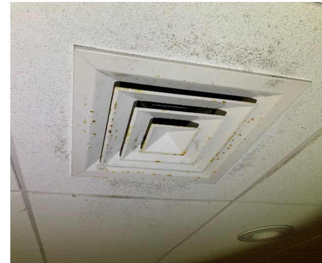
RUST AND CONDENSATION ON DIFFUSER
