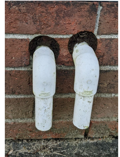
Missing Sealant & Wet Insulation
