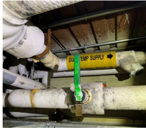
IMPROPER PIPE INSULATION
