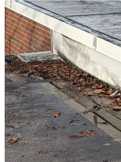
Failed Roof Membrane/ Ponding
