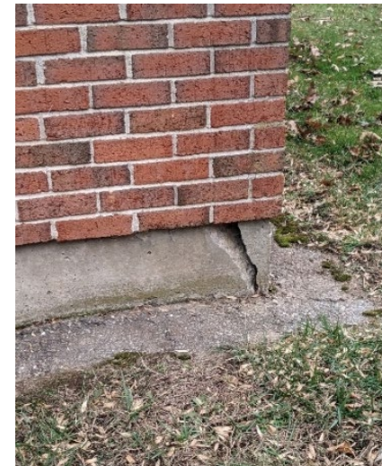
Cracked Foundation Wall
