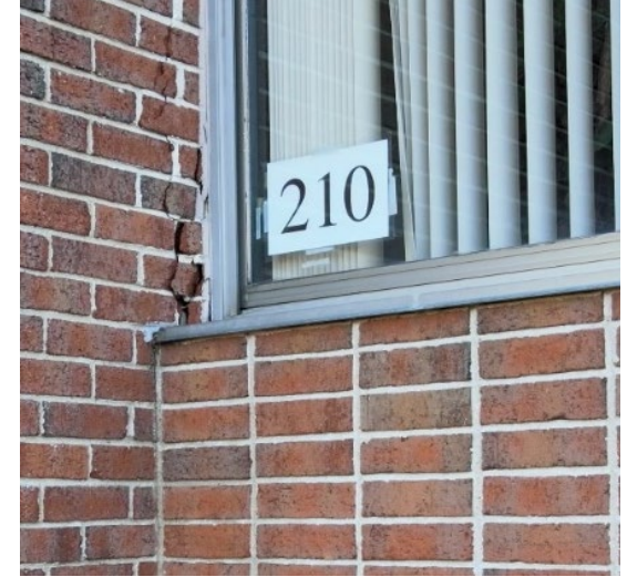
Cracking Masonry
