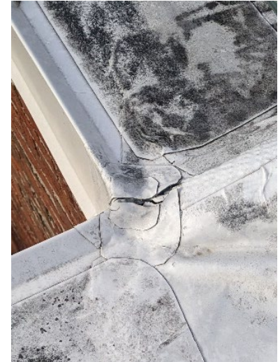
Failed Roof Membrane
