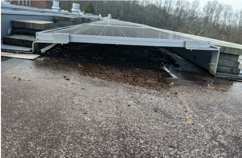
Water/ Debris Under Solar Panels
