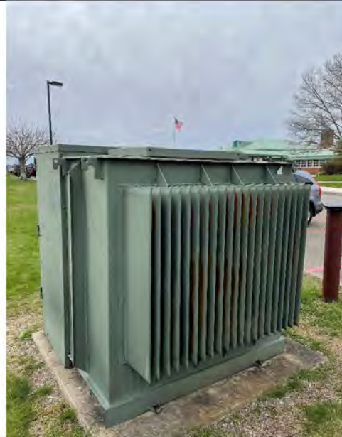
Photo # 27: - Utility Pad Mounted Transformer
