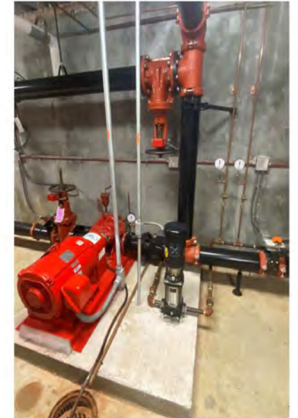
Photo # 68: Electric fire pump and jockey pump.
