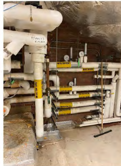
Photo # 3: Existing piping serving kitchen AHU
