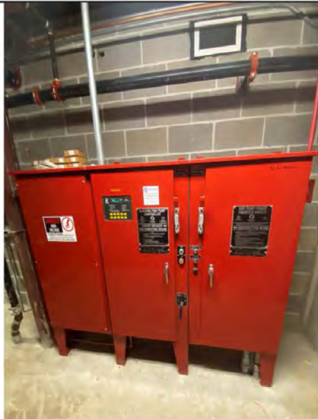
Photo # 55: - Fire Pump Controller
