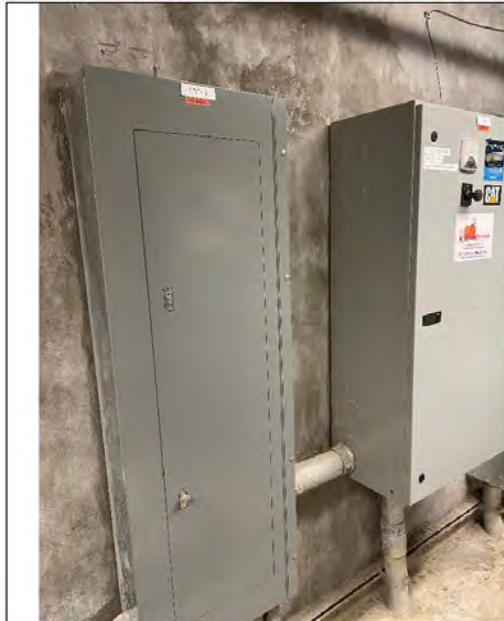
Photo # 37: - Life Safety Transfer Switch "ATS-1" and Distribution Panel "EDP-1"
