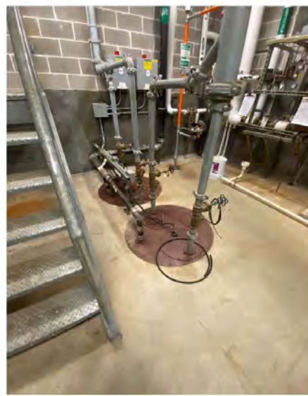
Photo # 24: Sump pumps located in domestic water pump room.
