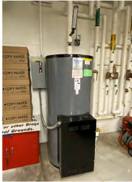
Photo # 1: Electric water heater with mixing valves.
