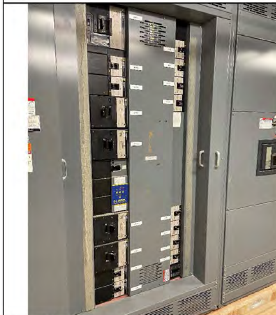
Photo # 31: - Switchboard "MSB-1" Distribution Section and Main Switch
