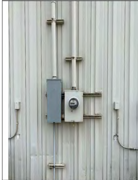
Photo # 67: - Utility Meter Socket and Tap Box
