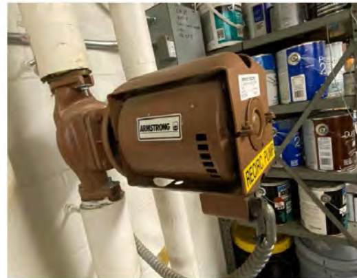
Photo # 3: Domestic hot water re-circulation pump.
