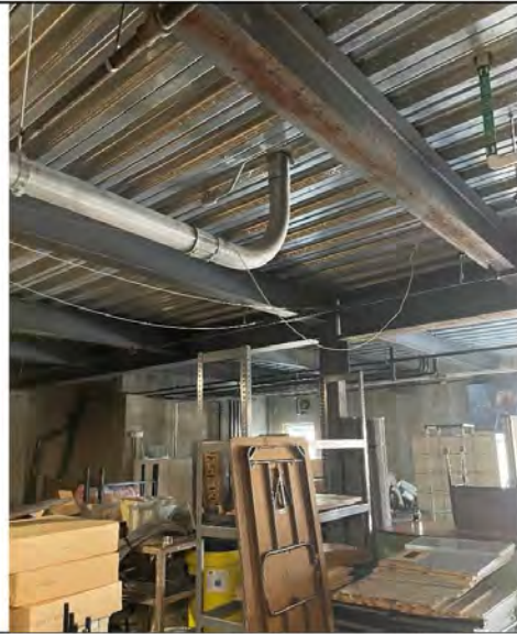
Photo # 34: - Conduit for Telecommunications Cabling up to Main Floor
