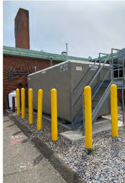
Photo # 9: Exterior, above grade, fuel oil tank
