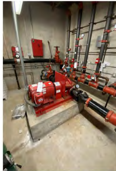
Photo # 11: Fire pump and sprinkler riser assembly.
