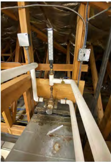
Photo # 8: Domestic water mixing valve.
