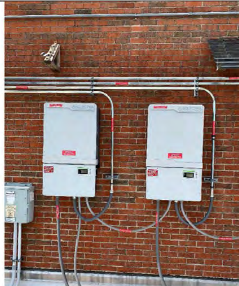
Photo # 40: - Typical Photovoltaic System Inverters on Roof
