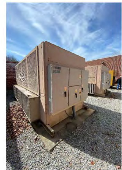
Photo # 12: Existing air cooled chillers.
