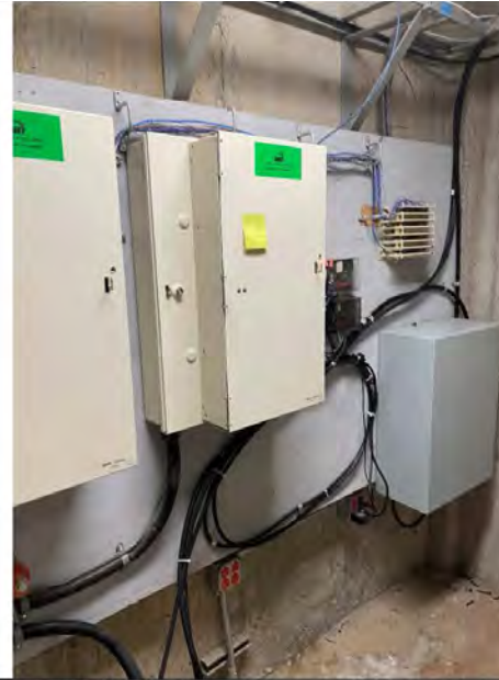
Photo # 57: - Main Telecommunications System Demarc
