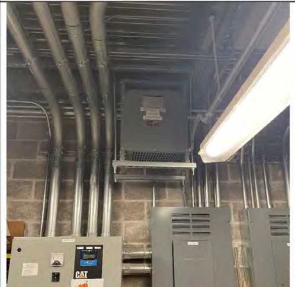
Photo # 36: - Standby ATS with Distribution Panel “ESB-1” and Transformer for Panel “EOP”
