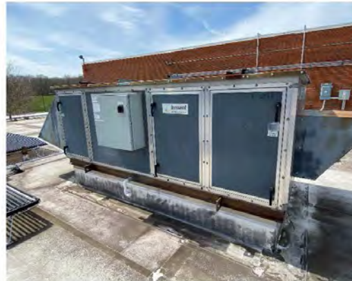
Photo # 19: Gas fired heat pumps- installed in 2017.
