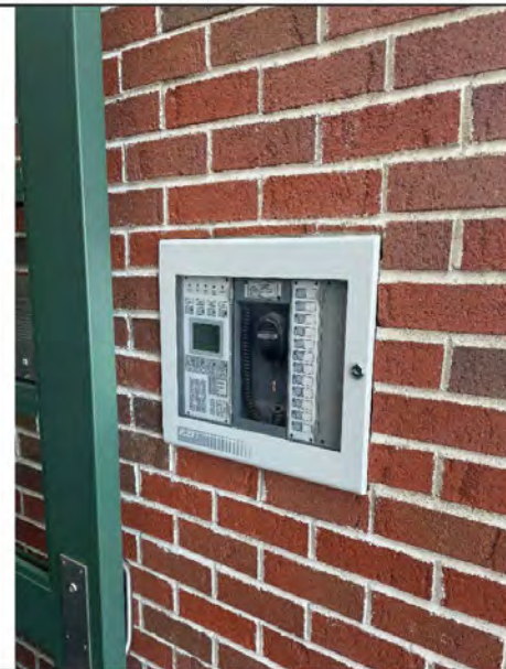
Photo # 51: - Fire Alarm Remote Annunciator Panel in Main Entrance Vestibule
