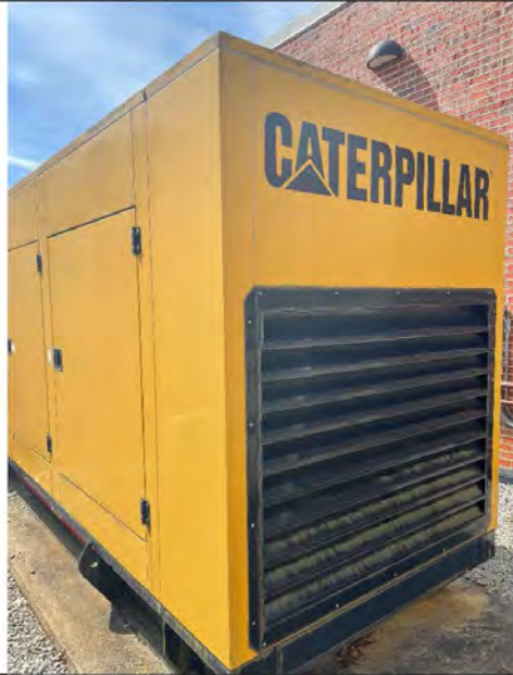
Photo # 37: - 400kW/500kVA Diesel Powered Generator with Sub-Base Fuel Tank
