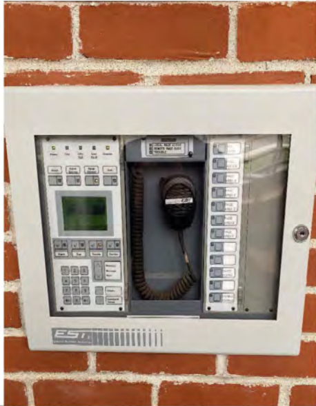
Photo # 53: - Typical Remote Annunciator Panel with Microphone for Voice Evacuation
