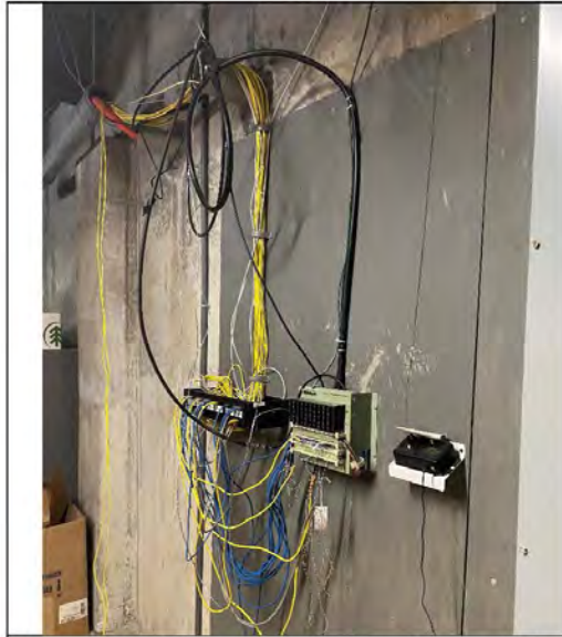
Photo # 33: Telecommunications Demarc with Fiber in Basement
