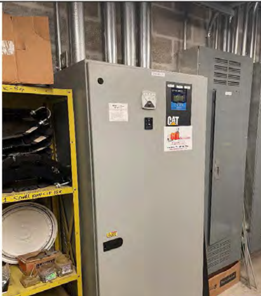
Photo # 35: - Automatic Transfer Switch – 600A (Optional Standby)
