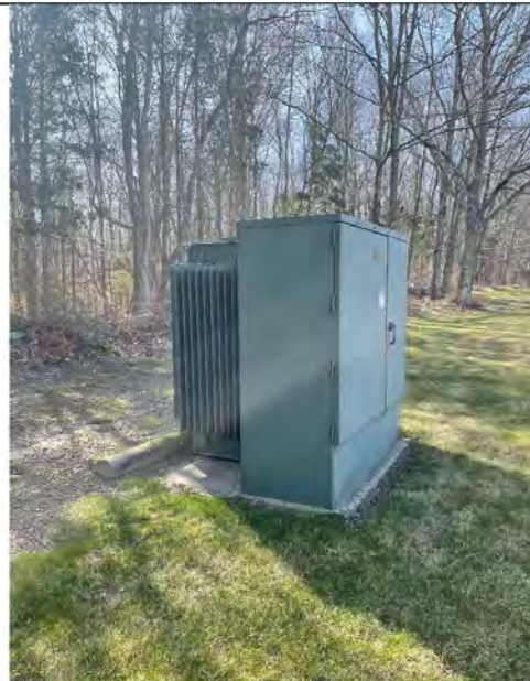
Photo # 27: - Utility Pad Mounted Transformer
