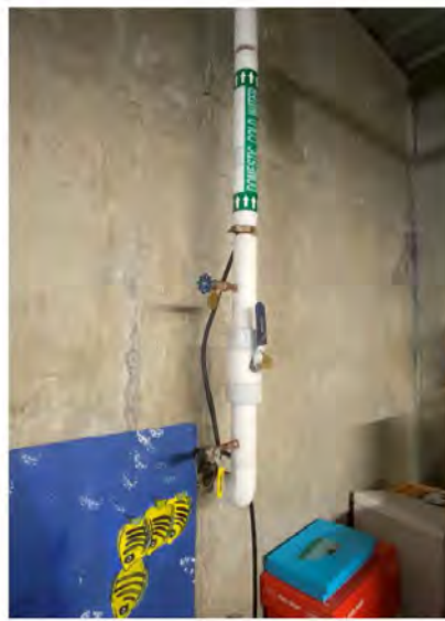
Photo # 12: Domestic water service entering through basement.
