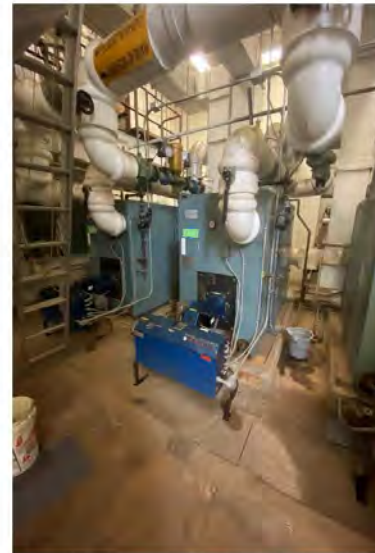
Photo # 11: Existing hot water boilers (Total of 3).
