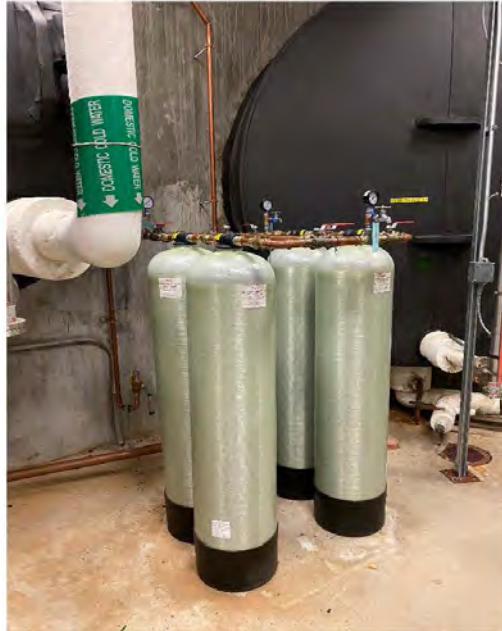
Photo # 22: Domestic water carbon filters
