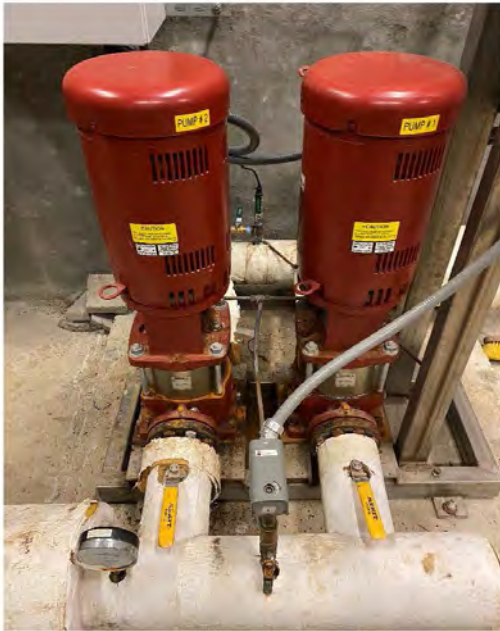
Photo # 21: Domestic water booster pumps.
