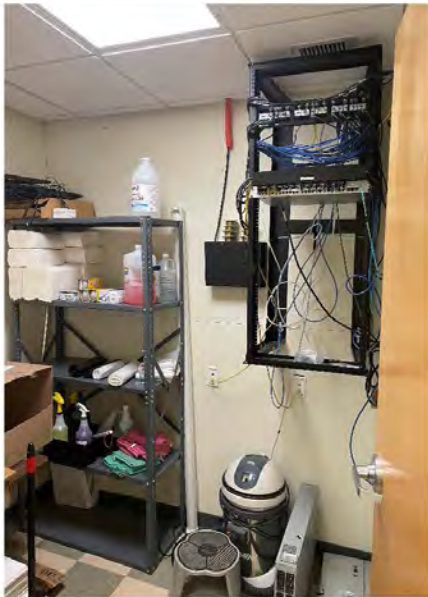
Photo # 35: - Telecommunications Rack with Fiber in Main Floor Storage Closet
