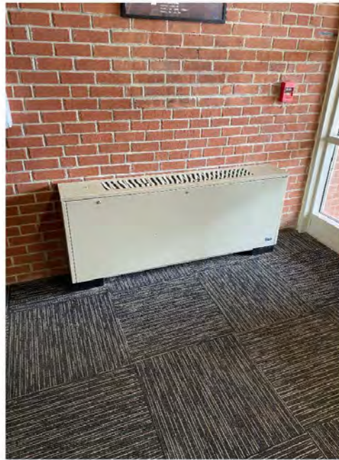
Photo # 5: Existing cabinet unit heater
