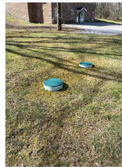
Photo # 16: Buried propane tank access covers.
