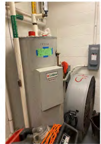
Photo # 74: Tech Ed: Existing electric domestic water heater.
