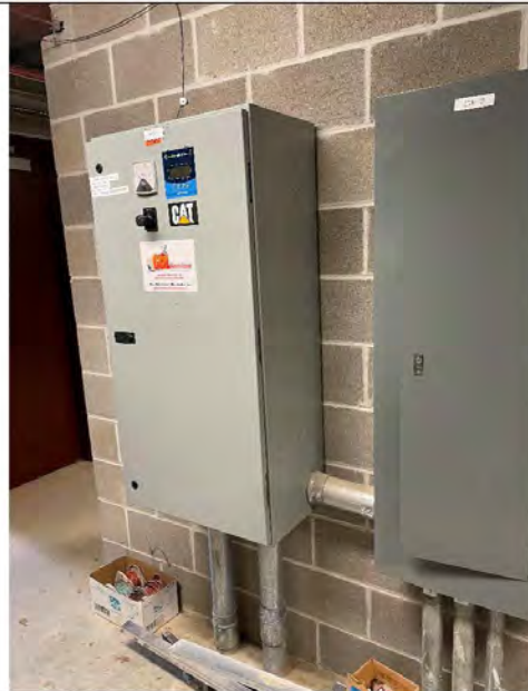
Photo # 38: - Standby Transfer Switch "ATS-2" and Distribution Panel "EDP-2"
