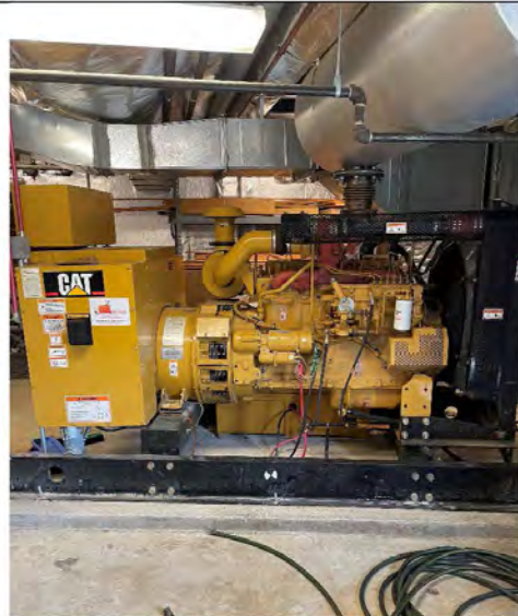
Photo # 40: - 250kVA/313kW Diesel Powered Generator
