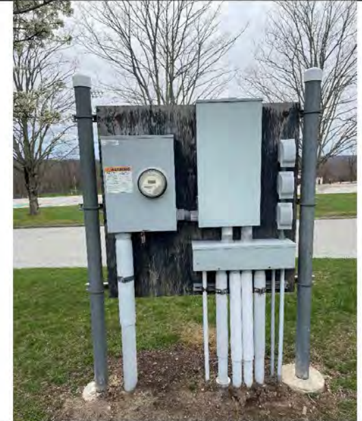
Photo # 28: - Utility Meter Cabinet with Tap Box and Feeders to Field House
