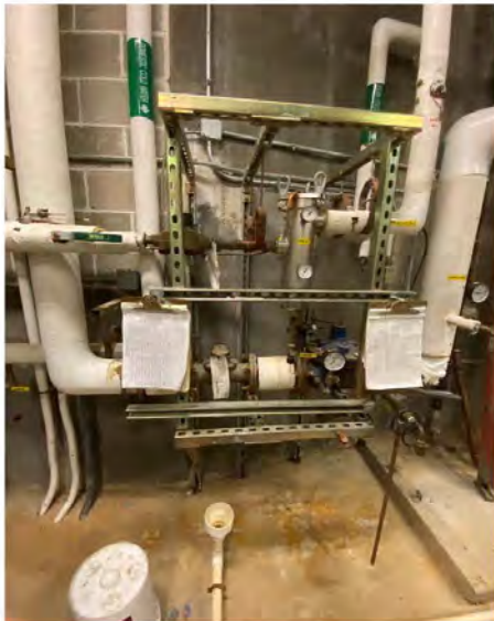
Photo # 23: Domestic water meter assemblies.
