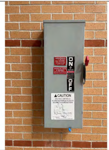
Photo # 42: - Photovoltaic System Main Disconnect and Meters
