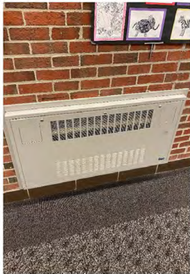
Photo # 15: Semi recessed cabinet unit heater.
