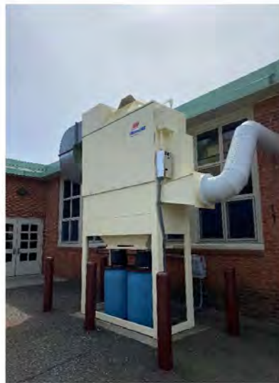
Photo # 8: Exterior dust collector serving wood shop classroom.
