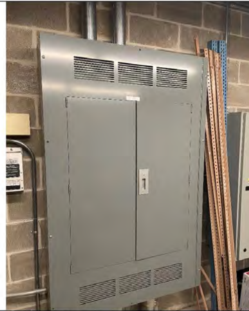
Photo # 33: - Emergency Distribution Panel “EDP”
