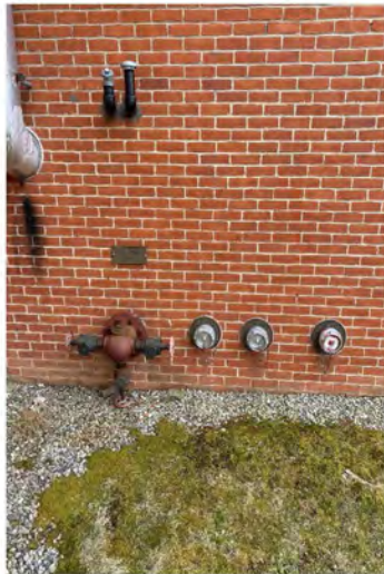
Photo # 71: Fire protection test header and fire department connection.
