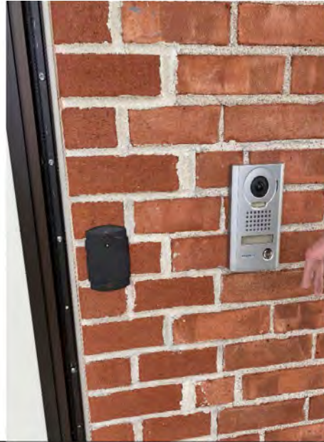
Photo # 62: - Card Reader and Aiphone Video Monitoring Station
