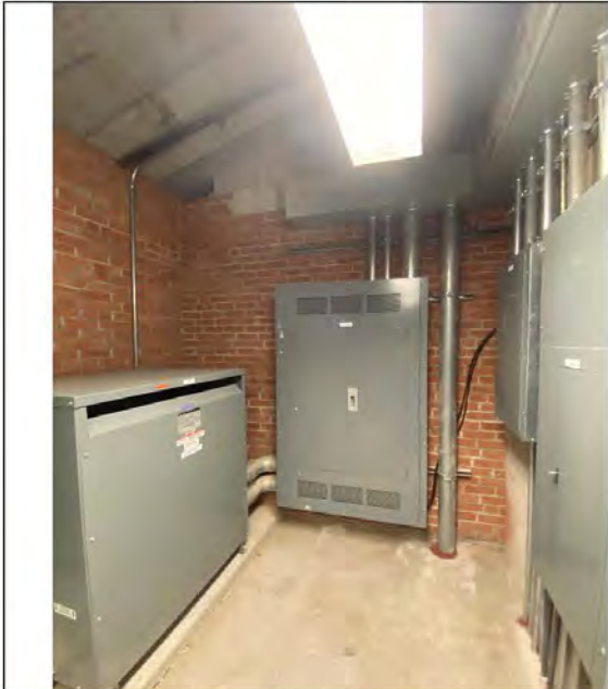
Photo # 33: - Transformer and Distribution Panels in Building Area "B"
