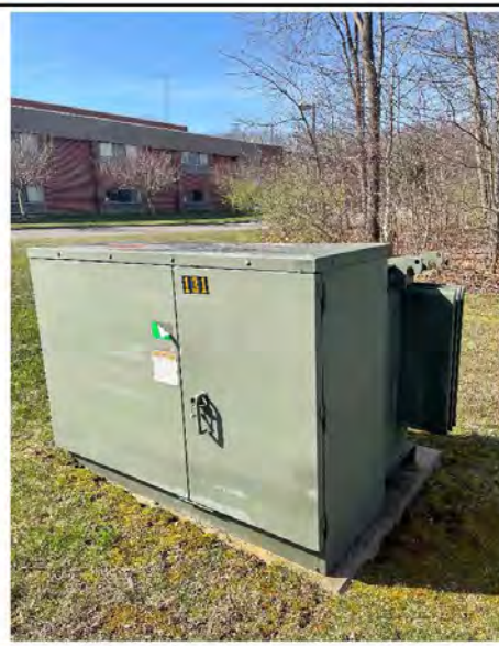
Photo # 18: - Utility Pad Mounted Transformer
