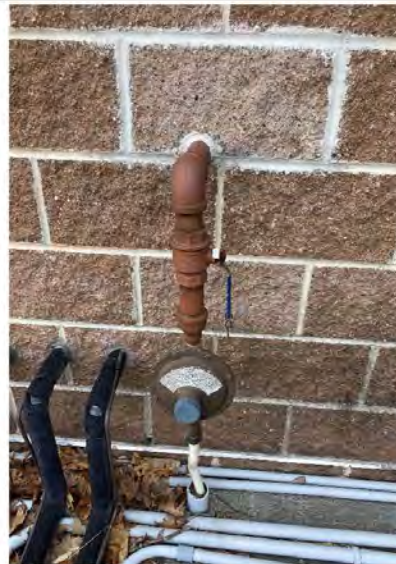
Photo # 15: Propane gas service into building.
