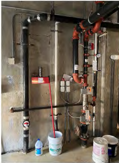
Photo # 11: Fire Protection service entering through basement.
