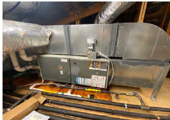
Photo # 4: Gas fire furnace located in attic space.
