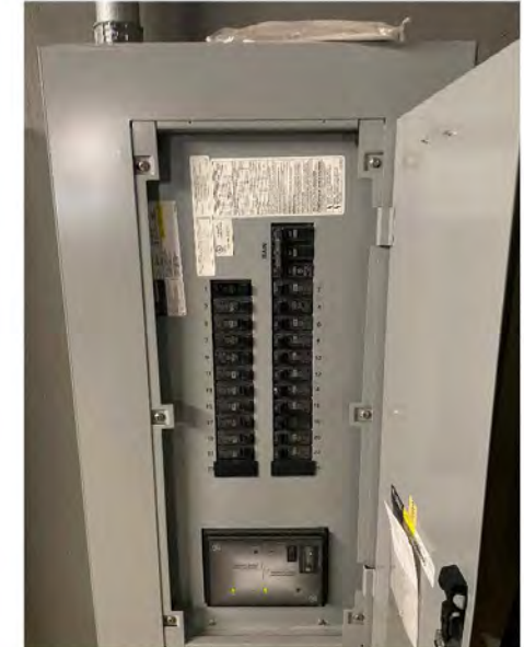
Photo # 24: - Branch Panelboard Interior
