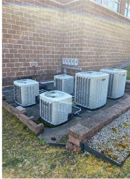
Photo # 10: Air cooled condensing units serving gas fired furnaces in attic space.
