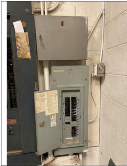
Photo # 69: - GE Load Center Panel
