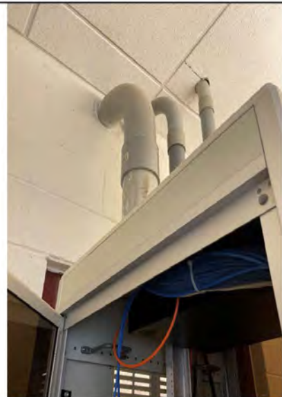
Photo # 72: - Telecommunications Conduits into Rack
