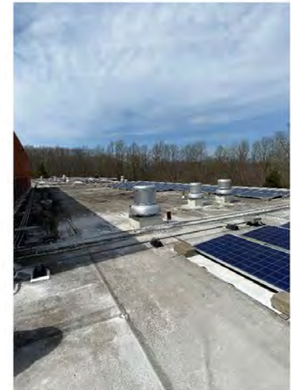
Photo # 20: Typical roof mounted exhaust fans.
