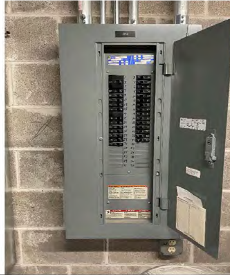
Photo # 30: - Typical "CP" for Mechanical Equipment
