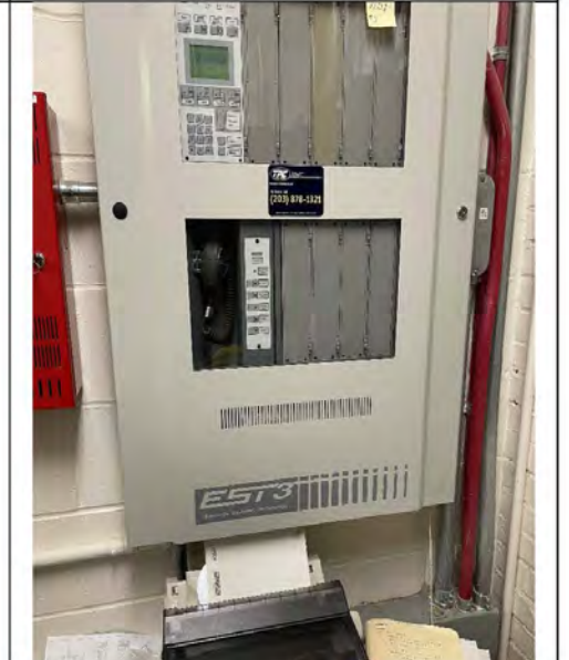
Photo # 52: - Typical Fire Alarm System Control Panel (one of three that serve the facility)
