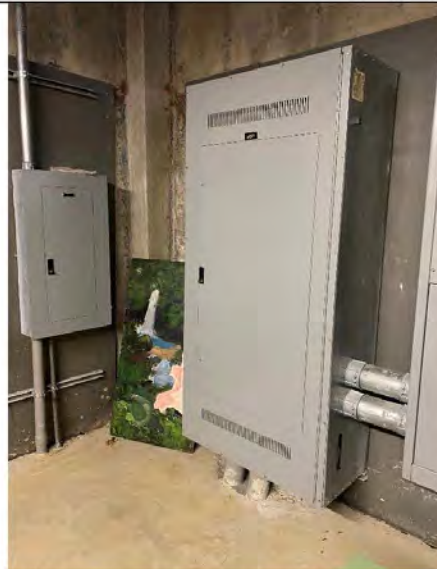
Photo # 21: - Service Entrance Equipment – Main Distribution Panel “MDP”
