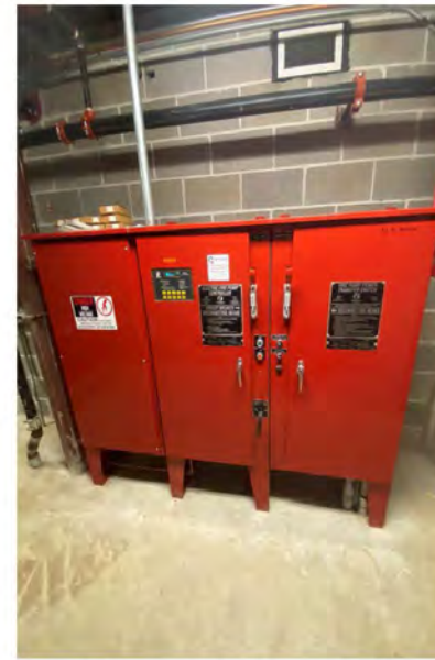
Photo # 67: Electric fire pump control panels.
