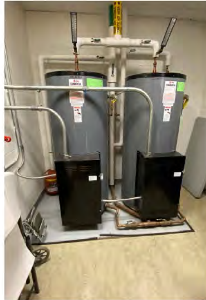
Photo # 14: Existing electric domestic water heaters.
