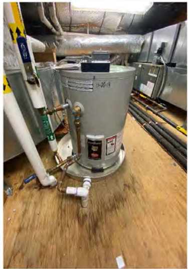
Photo # 7: Domestic hot water heater.
