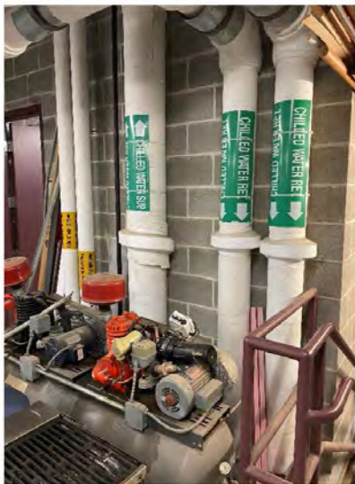
Photo # 7: Chilled water distribution piping.
