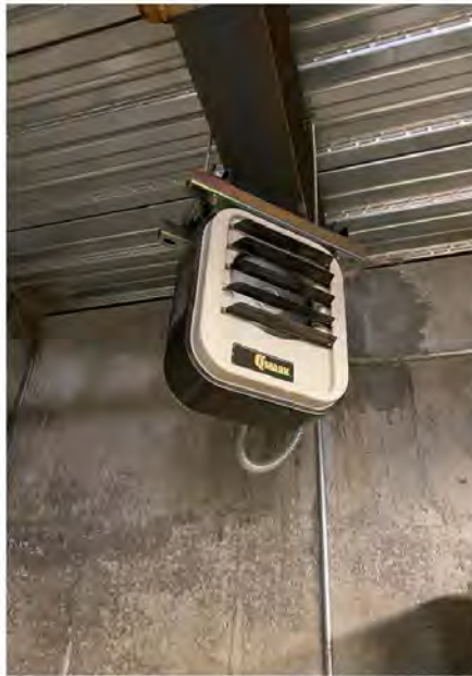
Photo # 13: Electric unit heater for freeze protection of basement area.
