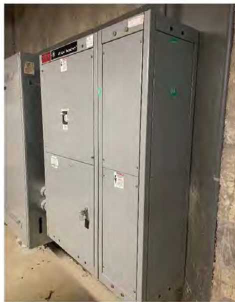
Photo # 20: - Service Entrance Main Switch and CT Cabinet in Basement
