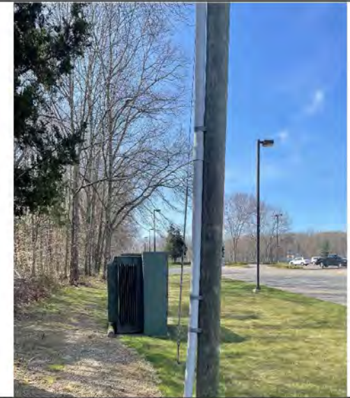
Photo # 26: - Utility Service Pole Primary and Telecommunications with Utility Transformer
