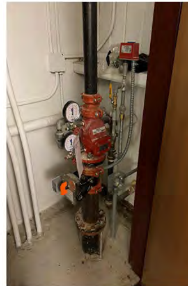
Photo # 75: Tech Ed: Fire Protection riser assembly.
