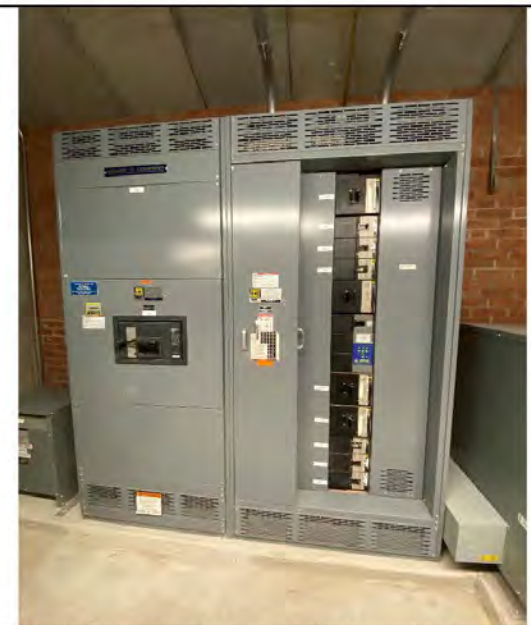
Photo # 32: - Distribution Switchboard "HBDB" in Building Area "B" Electrical Room
