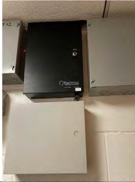
Photo # 61: - Access Control Headend Equipment (KerriSystems)
