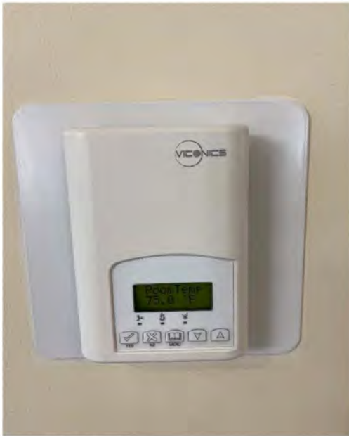
Photo # 1: Typical thermostat.
