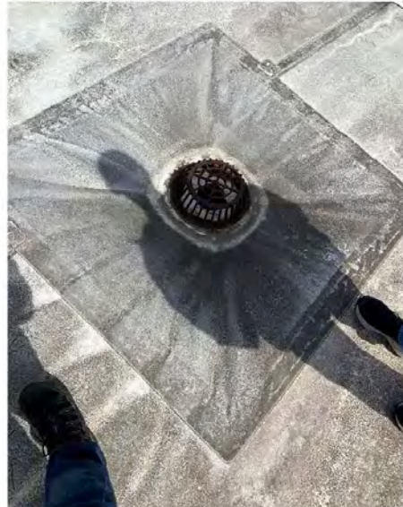
Photo # 24: Roof drain.
