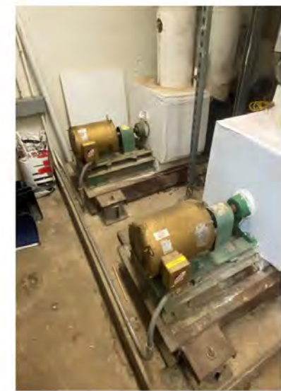
Photo # 12: Existing chilled water pumps
