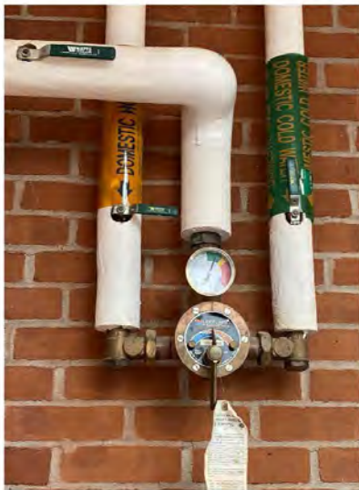
Photo # 7: Mixing valve serving emergency showers.
