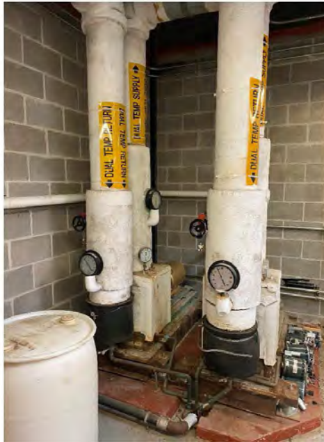
Photo # 5: Dual temp base mounted pumps.
