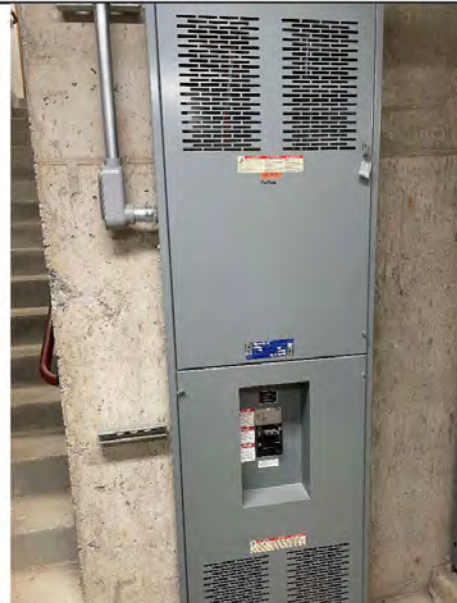
Photo # 56: - Fire Pump Disconnect
