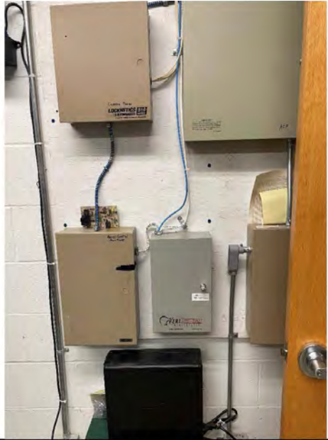
Photo # 58: - Access Control System Headend Equipment
