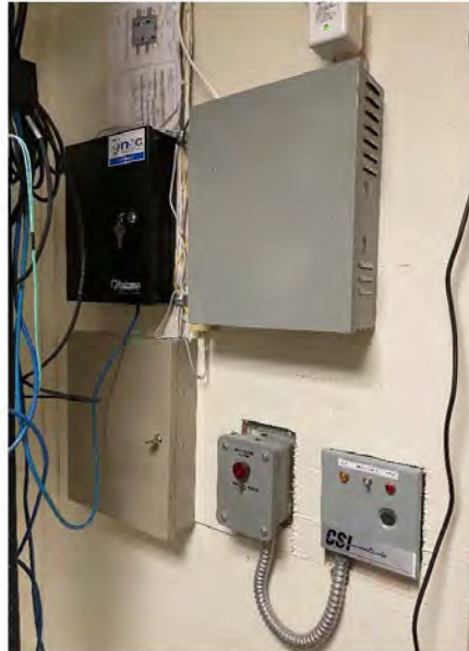
Photo # 36: - Security Access Headend Equipment
