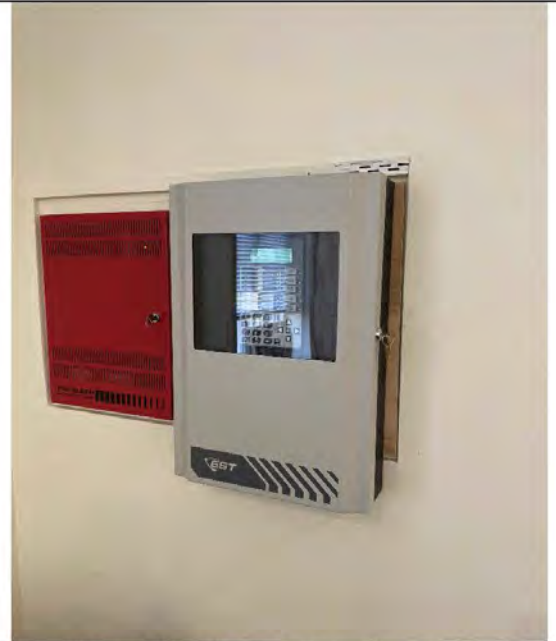
Photo # 30: - Fire Alarm Service Control Panel and Booster Cabinet at Main Entry
