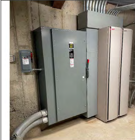
Photo # 35: - Disconnect for Theatrical Lighting and Dimming System Racks
