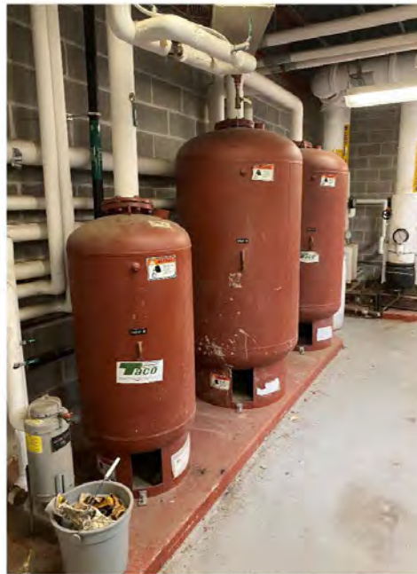
Photo # 6: Expansion tanks for hydronic systems.
