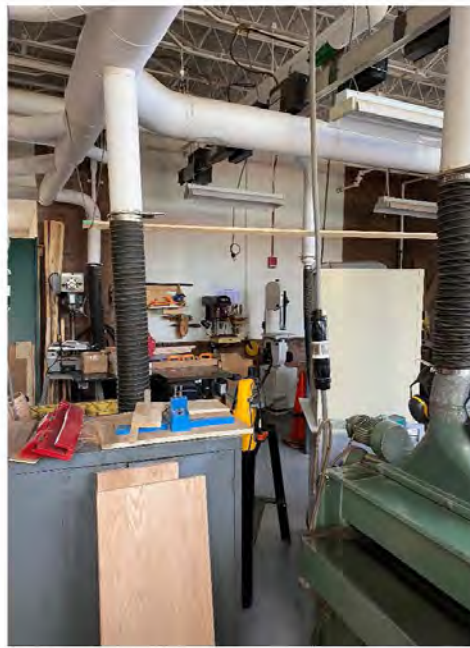
Photo # 6: Wood shop classroom with overhead ductwork to dust collector.
