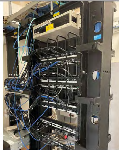
Photo # 59: - IDF Rack and Equipment (one of three that serve the facility)
