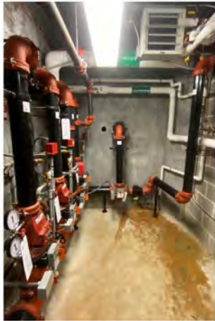
Photo # 69: Fire protection riser assemblies.
