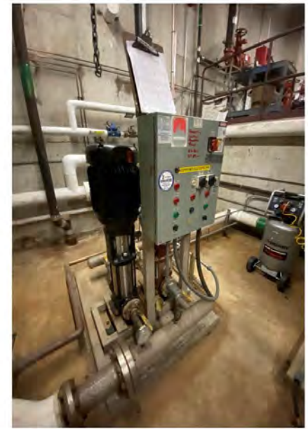
Photo # 10: Domestic water booster pump system.
